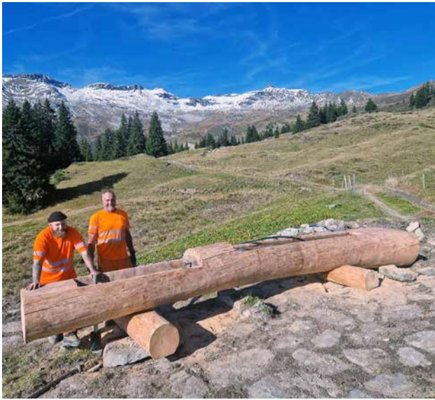
Installation Holzbrunnen Alp Ranasca
